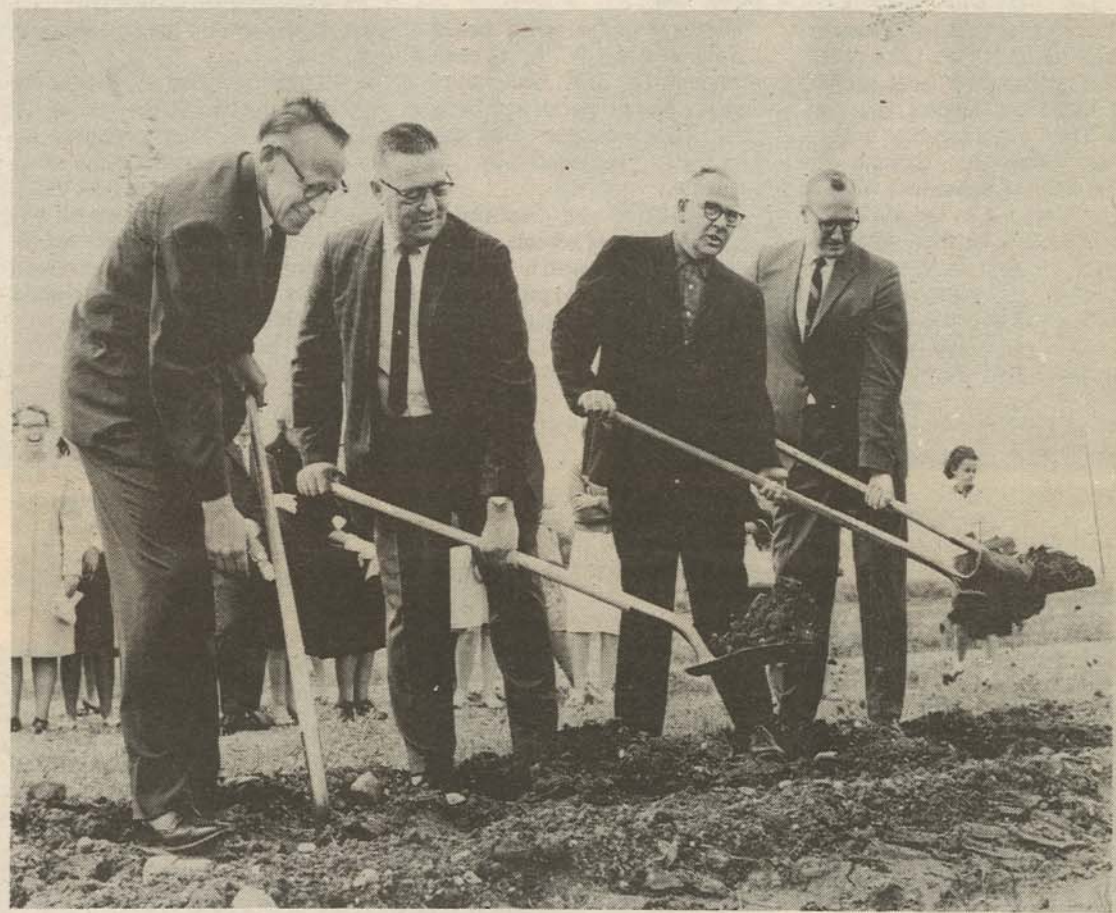
Turning the first shovels of dirt for construction of the new campus were, left to right, Merrill Berg, dean of the college; Clarence Erlandson, college president and superintendent of schools; Tom Goulding, president of the Devils Lake School Board, and William Bergstrom, president of the Community College Corporation.
